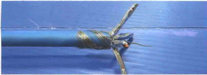
3. Spread apart the four pairs
